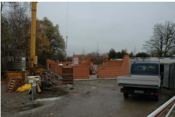
Pullinger Seen Baustelle Kiosk
